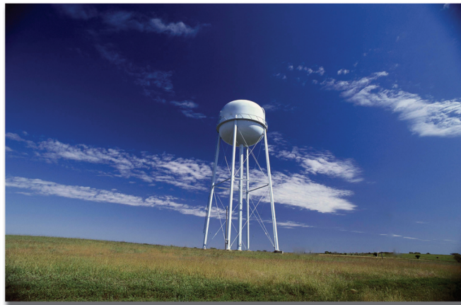
A new galvanic CP technology developed for water storage tanks like the one shown here uses power generated by magnesium anodes to operate a controller that automatically regulates tank-to-water voltage potential. Photo courtesy of Farwest Corrosion Control Co.
