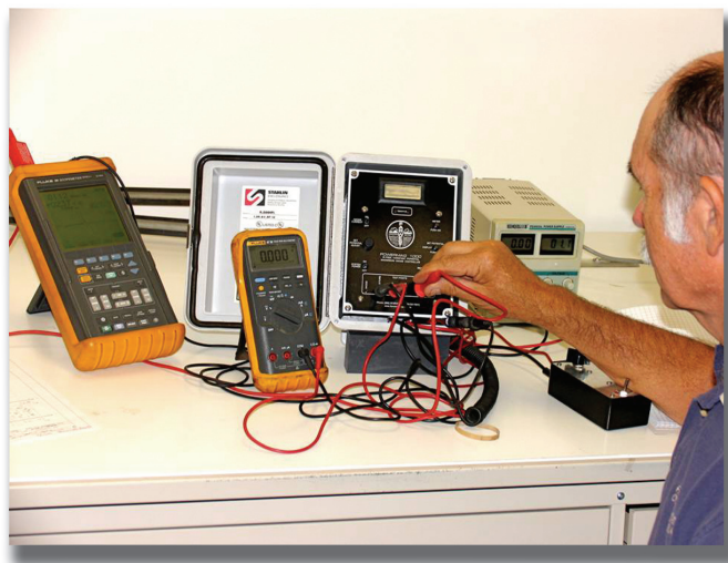
John Bollinger works on the controller system powered by a magnesium sacrificial anode-cathode cell. Photo courtesy of Farwest Corrosion Control Co.
