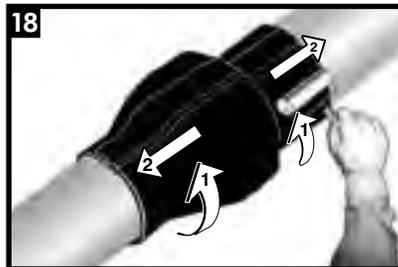
While the sleeve is still hot and soft, use a hand roller to firmly roll the sleeve surface and push any trapped air up and out of the sleeve, as shown above. If necessary, reheat to roll out air.
