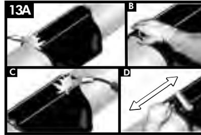
Gently heat the closure and pat it down with a gloved hand. Repeating this procedure, move from one side to the other. Smooth any wrinkles by gently working them outward from the centre of the closure with a roller.
