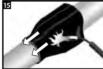
Continue shrinking from the bell of the tyton joint to the sleeve end. Sleeve recovery is complete when it conforms to the pipe.
