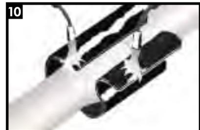
Wrap the WLOX sleeve around the tyton joint. Gently heat the backing of the underlap and the adhesive side of the overlap. Finish wrapping the sleeve around the tyton joint pressing the overlap firmly into place.
