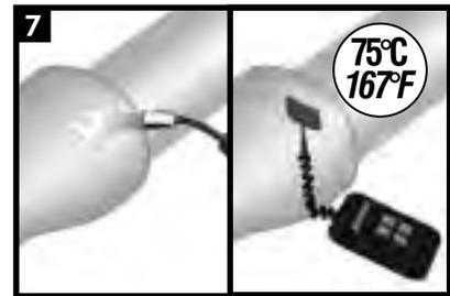
Pre-heat the joint area to a minimum of 75°C (167°F). Using a temperature measuring device, ensure that the correct temperature is reached on the steel and at least 50 mm (2") on each side of the sleeve.
