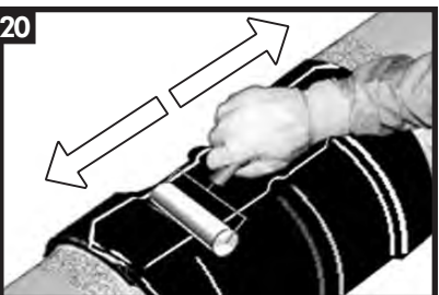
Continue the procedure by also firmly rolling the closure with long horizontal strokes from the weld outwards.
