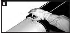
Gently heat the closure and pat it down with a gloved hand. Repeating this procedure, move from one side to the other. Smooth any wrinkles by gently working them outward from the centre of the closure with a roller.
