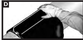
Gently heat the closure and pat it down with a gloved hand. Repeating this procedure, move from one side to the other. Smooth any wrinkles by gently working them outward from the centre of the closure with a roller.
