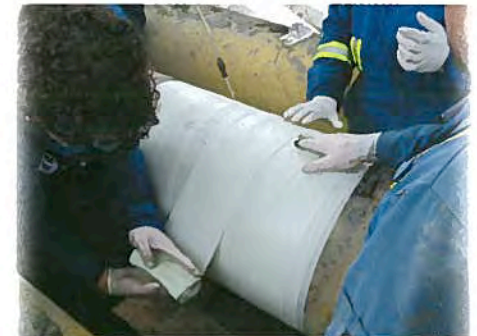
2 Wrap Syntho-Glass over Petroleum Tape
