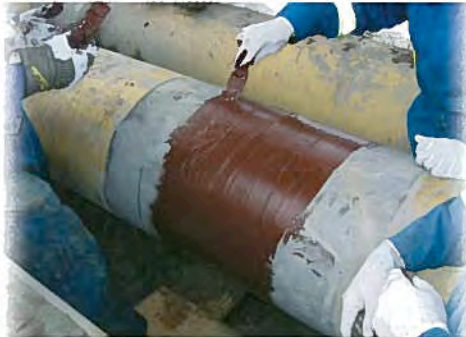
1 Apply 2-part Syntho-Steel Epoxy
