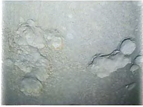
Corrosion damage on 10" pipe
