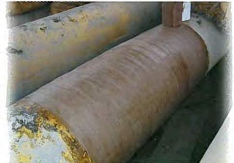
1 Wrap Petroleum Tape over area to protect
