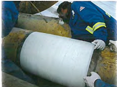
3 30 Minutes later, project complete
