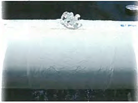
1 inch by 1/4 inch crack in pipe
