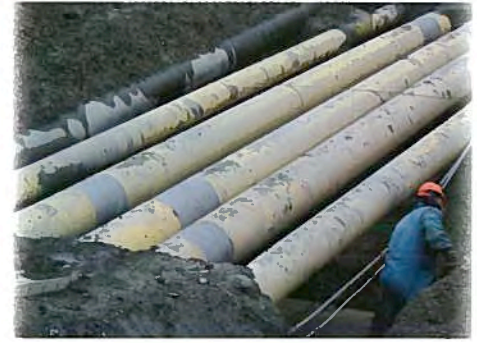
Potential corrosion area on pipeline
