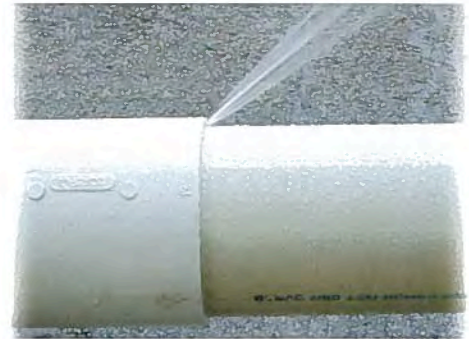
Leaking joint on a 4" line
