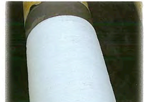
3 In 30 minutes, material is set and ready for back fill.
