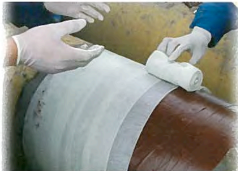
2 Syntho-Glass® wrapped over Epoxy
