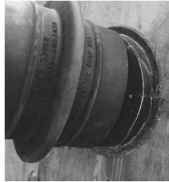
3. Place the Century-Line® Sleeve on the end cap. The sleeve and endcaps total length should be one-fourth longer than the width of the wall. Cut with a hand or power saw.
