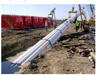
In September of 2009 an engineering firm in charge of the design for this directional drilling project contacted Jim Tolly, Technical Sales Representative for Corrosion Control Products Company, for assistance. The project consisted of 10 bundled casings, including  $3-14^{\circ}$ ,  $2-12^{\circ}$ ,  $2-10^{\circ}$ ,  $1-6^{\circ}$ , and  $2-4^{\circ}$  pipe casings. The client was interested in coating options for the girth welds along the various casings.
