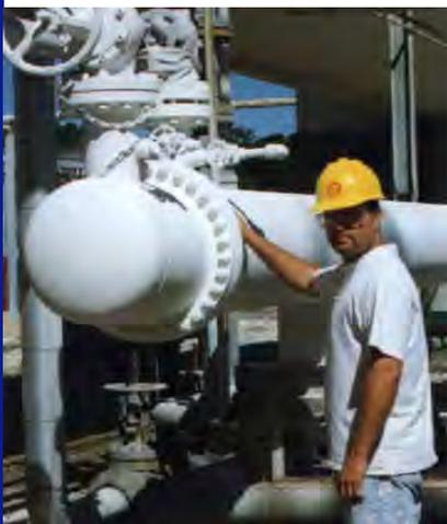
Mascoat has recently proven, in a study presented to NACE, that its hallmark thermal insulating coating, Industrial-DTI, is capable of protecting personnel from burns up to 375°F (190°C) to ASTM C1055 & C1057 standards. Anyone who has touched a DTI coated surface knows that they can keep their hand on it much longer than the required 5 seconds.
