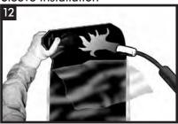
Partially remove the release liner and gently heat the underlap approximately 150 mm (6") from the edge.
