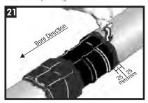
Apply epoxy to trailing edge of first sleeve; 25mm (1") onto sleeve, 25mm (1") onto adjacent coating. Epoxy applied should thoroughly cover the edge of the sleeves. It is best to allow the epoxy to cure at ambient temperature. If necessary, use a low flame to cure epoxy. Cover the entire sleeve with any left-over epoxy.
