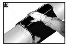
Press the closure firmly into place. Gently heat the closure and pat it down with a gloved hand. Repeating this procedure, move from one side to the other. Smooth any wrinkles by gently working them outward from the centre of the closure with a roller.
