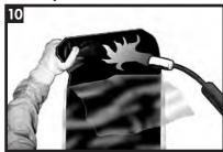
Using the wider sleeve, partially remove the release liner and gently heat the underlap approximately 150 mm (6") from the edge.
