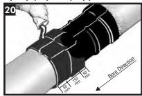
When the sleeve is between 15 - 40°C, apply epoxy over the sacrificial sleeve to form a wear cone; covering 50mm (2") onto the pipe coating, the entire sacrificial sleeve and 50mm (2") onto the first sleeve. Epoxy applied should thoroughly cover the edge of the sleeves.
