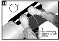
Centre the sleeve over the joint so that the sleeve overlaps between the 10 and 2 o'clock positions. Press the underlap firmly into place. Remove the remaining release liner.
