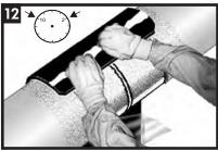
Centre the sleeve over the joint so that the sleeve overlaps between the 10 and 2 o'clock positions. Press the underlap firmly into place and remove the remaining release liner.
