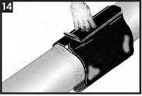
Remove any release liners from the Closure Strip . Centre the closure on the overlapping sleeve. Press down firmly.
