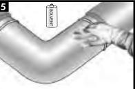
Ensure that the PE coating edges are beveled to 30°. Clean exposed steel and adjacent pipe coating with a solvent cleanser to remove the presence of oil, grease, and other contaminants.
