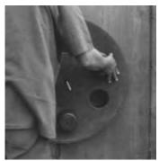
**3.** Slide the first Cell-Cast<sup>®</sup> disk over the threaded rod.
