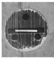
8. After wall cures, wall forms are removed. The Cell-Cast® disk assembly is now ready for removal.
