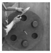
**4.** Secure the edges of the cell to the form using the provided steel spikes.
