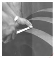
**5.** Additional disks are interlocked to accommodate finished wall thickness. Verify thickness is the same as wall.
