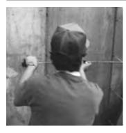
1. Locate center line where the hole is desired. This location will be used as a guide for the threaded centering assist rod.
