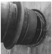
3. Place the Century-Line® Sleeve on the end cap. The sleeve and endcaps total length should be one-fourth longer than the width of the wall. Cut with a hand or power
