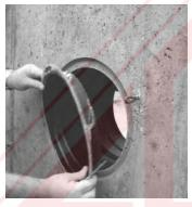
6. After the concrete is poured and cured, remove end caps with screw driver or crow bar. End caps may be replaced to protect sleeve until pipe penetration is made.
