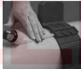
7B. Re-insert Slide-Locks completely into segments or until tight by driving Slide-Lock back into position while holding the Slide-Lock against the pipe.
