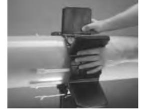
5. Align the buckles and lock into place. Take the final Slide-Lock and slide completely into place.
