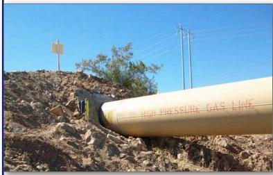
properly designed AC mitigation system. A C mitigation system. A C mitigation systems help to equalize the potential between the pipeline or structure and the local soil surfaces. Although the voltage is still present, the shock hazard (or 'touch potential') is greatly reduced.
