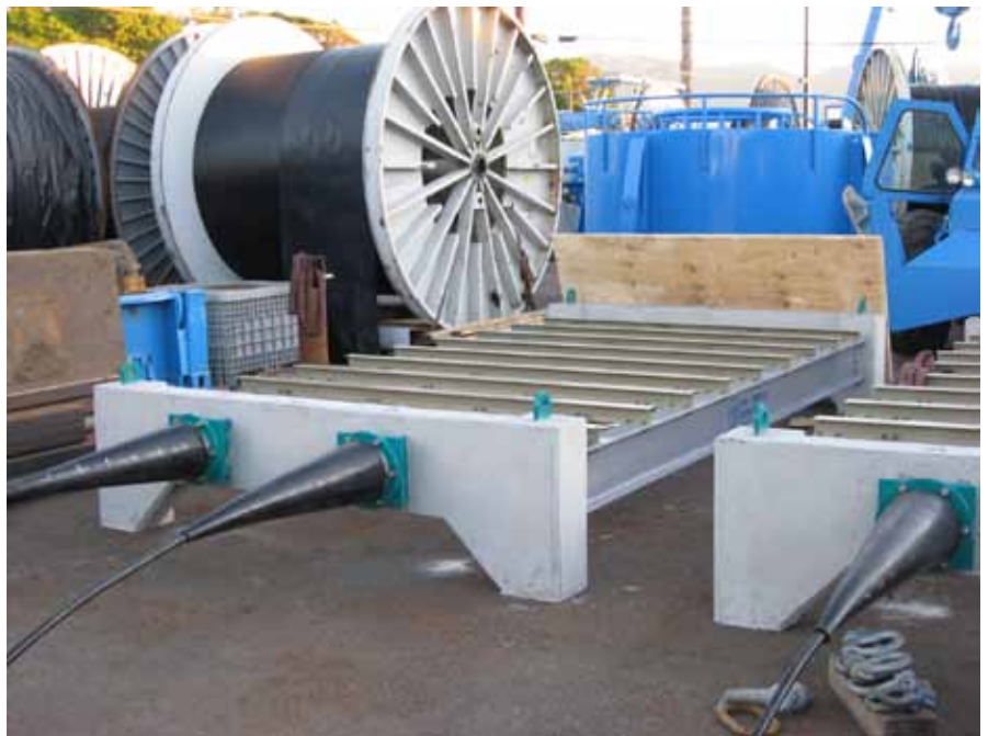
Shown is the completed anode sled. Photo courtesy of John Bollinger, Farwest Corrosion Control.
