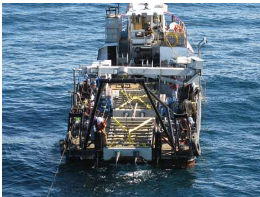
The boat crew prepares to install the first anode sled. Photo courtesy of John Bollinger, Farwest Corrosion Control Co.
