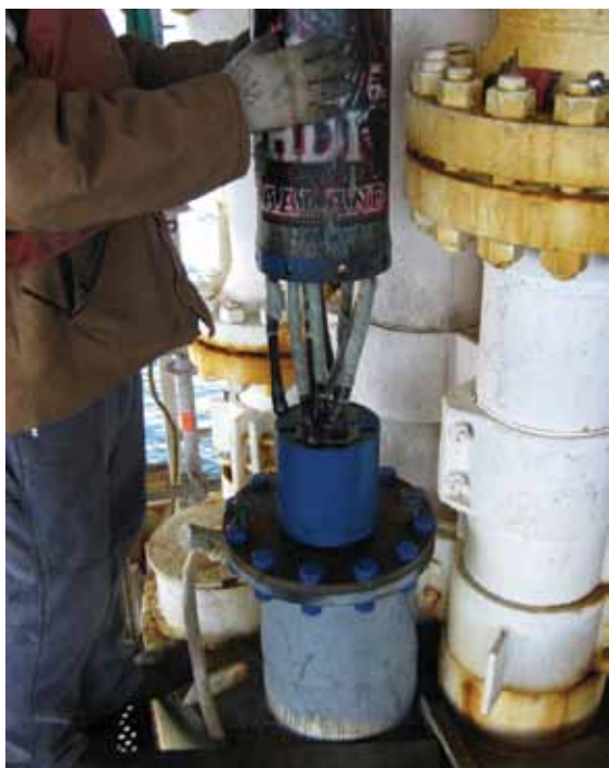
The pulling head is removed from the anode cable ends at the top of the J-tube aboard the platform. Photo courtesy of John Bollinger, Farwest Corrosion Control.
