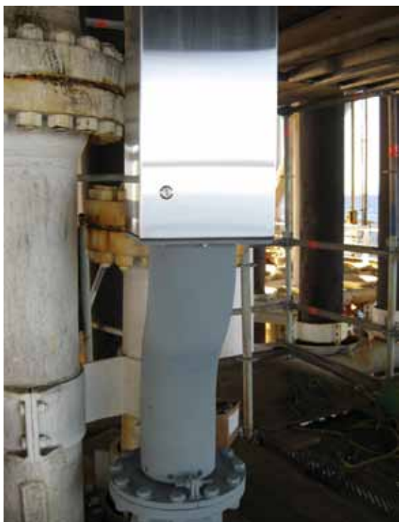
The cables from the newly installed anode sleds will be routed from the J-box to one of the platform's rectifiers. Photo courtesy of John Bollinger, Farwest Corrosion Control.
