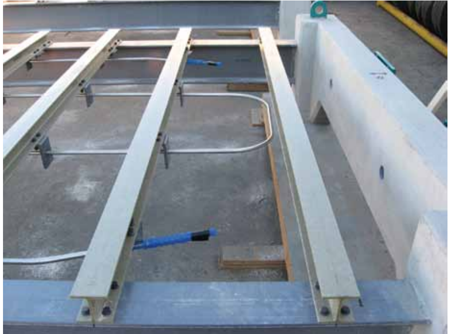
To fit the 50-ft platinum-clad anode rod into a compact sled, it had to be carefully formed into a modified "U" shape. Photo courtesy of John Bollinger, Farwest Corrosion Control.
