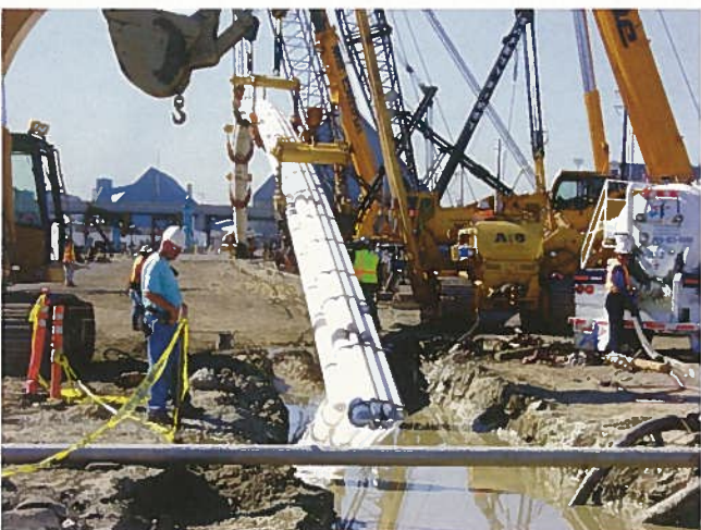
Figure 3. Rock, shale, and gravel can cut through or abrade coatings all the way to the pipe surface.
