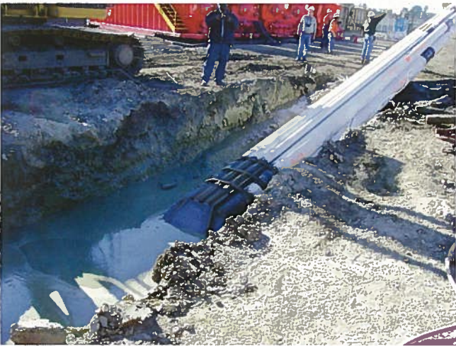
Figure 2. Coatings used in directional drilling projects are typically sturdier and more abrasion resistant than those used in direct bury applications.
