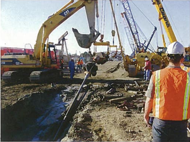
Figure 1. Pipelines pulled through the bore of a directional drill are subjected to stresses that can very easily damage or destroy their protective coatings.
