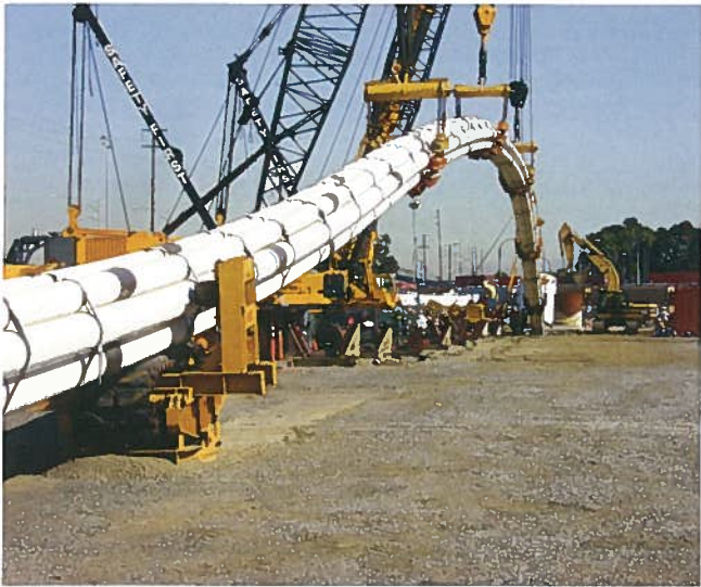
Figure 5. Pulling bundled casings.
