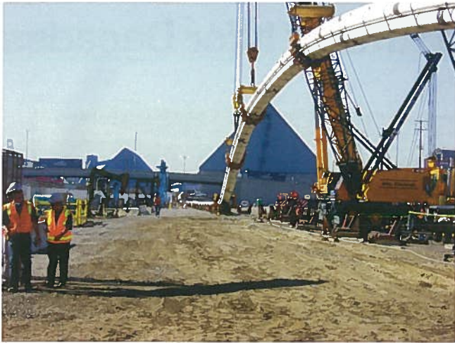
Figure 4. There are a multitude of field-applied girth weld coatings available for use in directional drilling projects.
