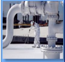
insulating and corrosion barrier for a variety of above ground applications. These include piping, storage tanks, process equipment, heat exchanges, and more. Applied directly to many substrates (requires a primer on steel), these insulating coatings help solve problems such as condensation build-up, corrosion under insulation (CUI), personnel burns, and energy loss. Products are easily applied via airless sprayer and clean-up is achieved with soap and water.
