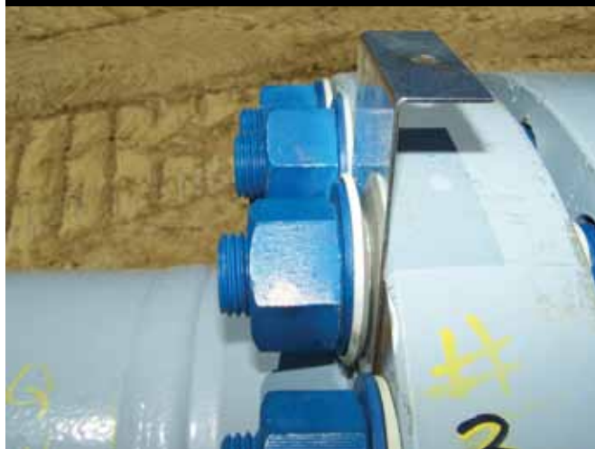
Over-compressed white isolation washer.
