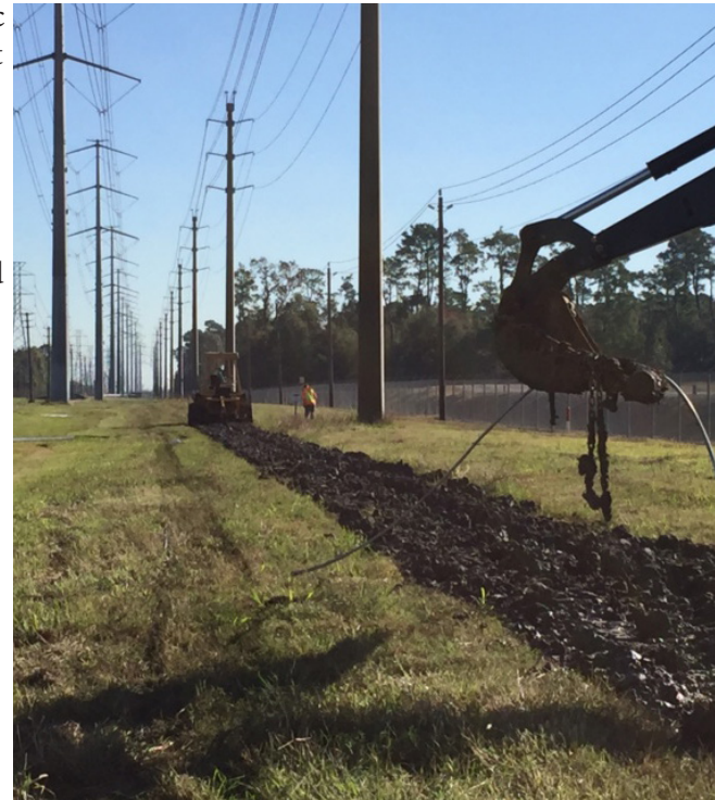
Figure 1 – Plattline used for AC mitigation
